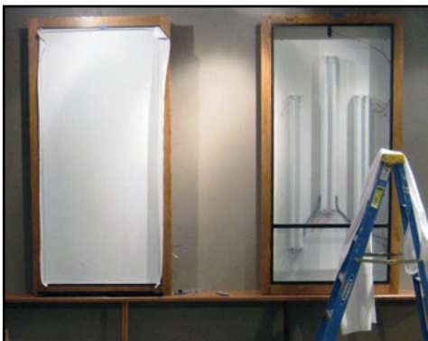
Light boxes for Lourdes Chapel, Cedar Lake, IN. On the left, diffusion fabric has been stretched and attached to the F channel.
