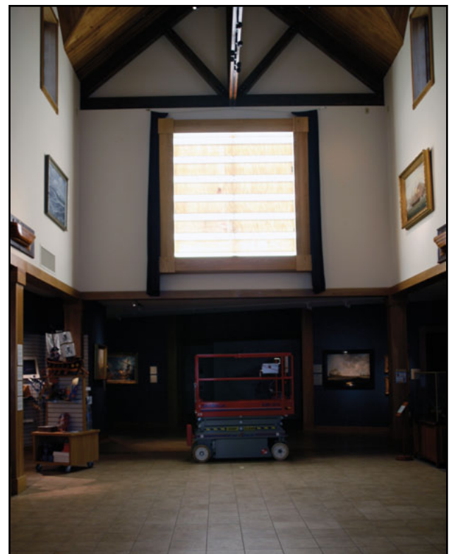
The light box for the MacKay window features UV covered fluorescent bulbs and access panels with piano hinges on the left and right of the box.
